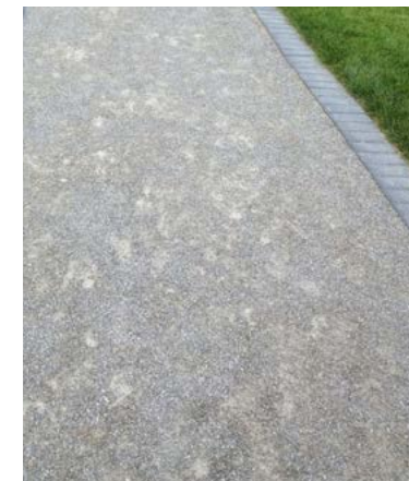
halfverharding in grind
